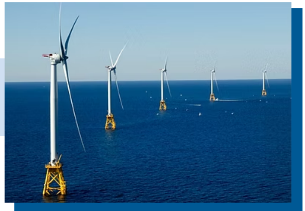
Block Island Wind Farm (Compliments E.W. Audet & Sons)
